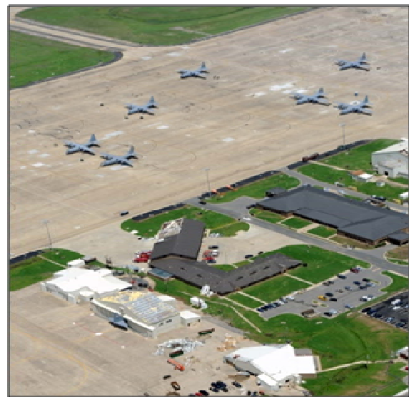
2011 Tornado Damage to Little Rock Air Force Base
