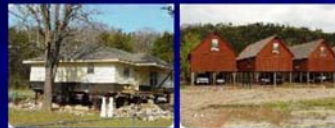
Crawford County, AR • Elevation Project Baxter County, AR • Elevation and tie-down
