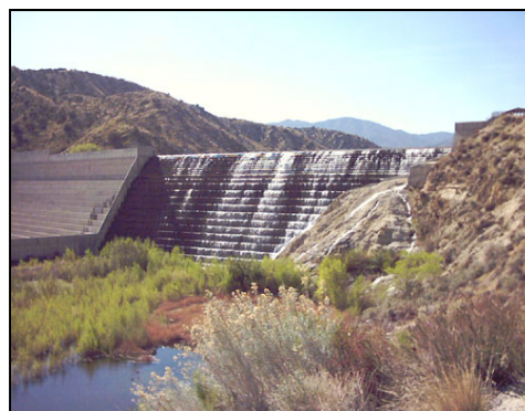
Little Rock Dam and Recreational Area
